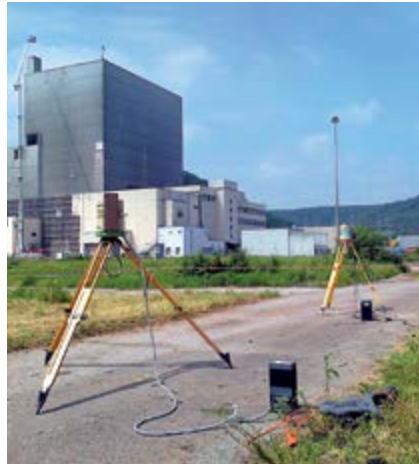
Control measurements in the area of nuclear plants
