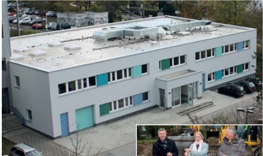
No more long distances: the new building for dosimetry in Dortmund.
