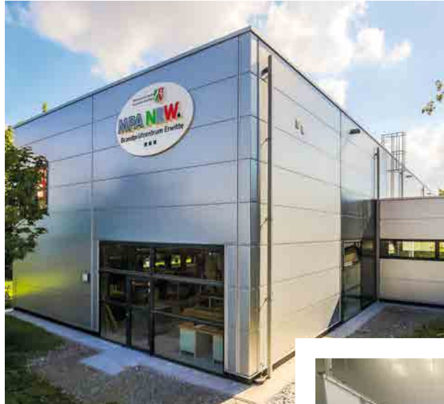
The new testing hall of the fire testing centre Erwitte.
